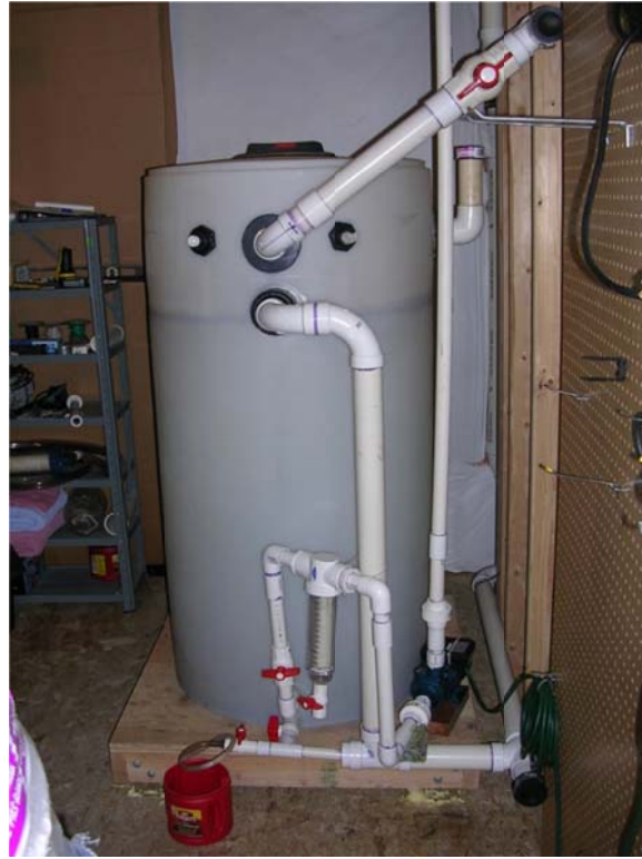
Figure 2-3. Graywater Storage Tank at Existing Household in Fort Collins, CO (existing system). Photo by J. Bergdolt.
