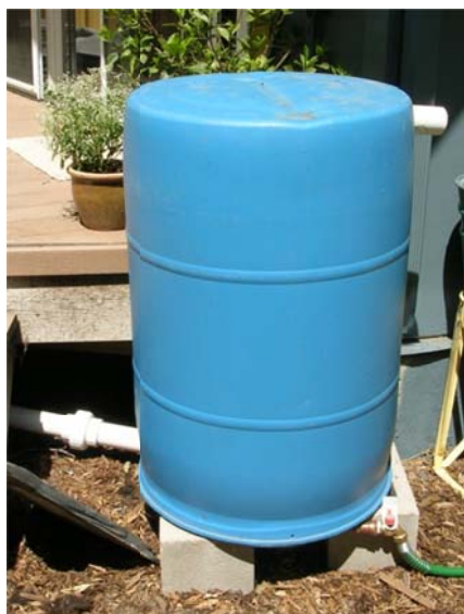
Figure 2-7. Outdoor Storage Tank with Gravity Feed of Graywater Through Hose in Fort Collins, CO (new installation).
