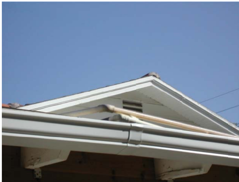
Figure 2-5. Graywater Pipes to Gutter for Irrigation in Phoenix, AZ (new installation).
