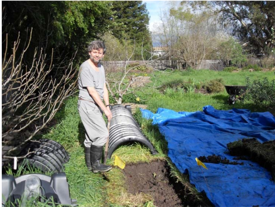
Figure 2-6. Subsurface Infiltration of Graywater in Cotati, CA (new installation).
